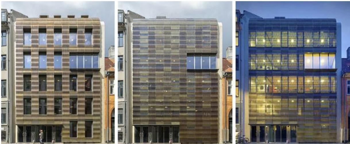
The design is defined by a patterned, perforated golden copper alloy curtain, incorporating motorized folding elements, that effectively changes the architecture of the building. The judges said: *"This transformable building is a unique and powerful response to its urban context – surprising, yet obvious. The central concept is carried through undiluted and executed with care to an impressive level of detail."*
